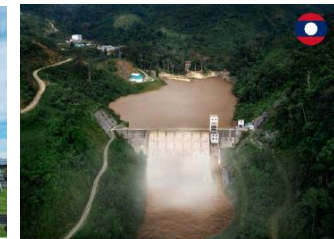
Hydro Power (2 Sites)
